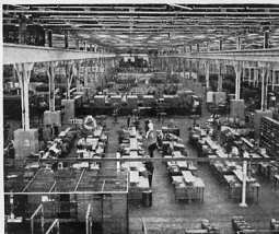
An interior view of just one section of the famous Willow Run bomber plant, one of the largest and finest factories in the world, which is now being converted for the mass production of new and advanced automobiles and modern farm equipment.
